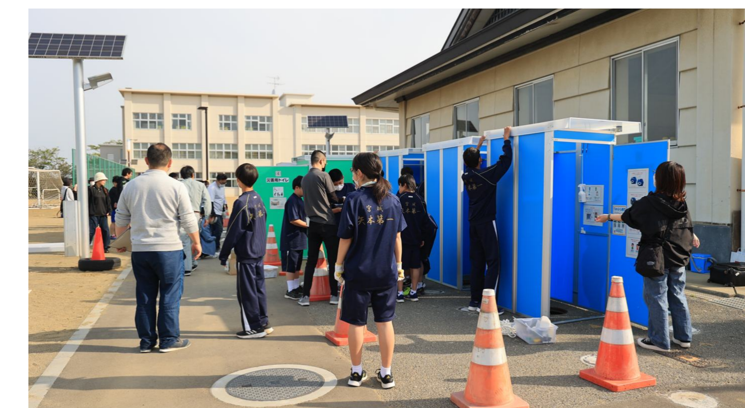
早朝から先生や生徒、保護者が集まり自分たちで組立てる Teachers, students and parents are setting up manhole toilets.
